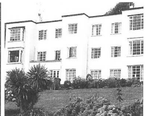
When replacing windows match the glazing pattern to suit the period of the property. Horizontal glazing patterns are typical of the interwar period.
