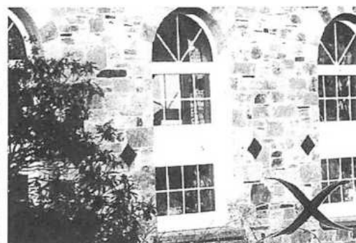
Avoid incorrectly detailed fan-headed windows.
