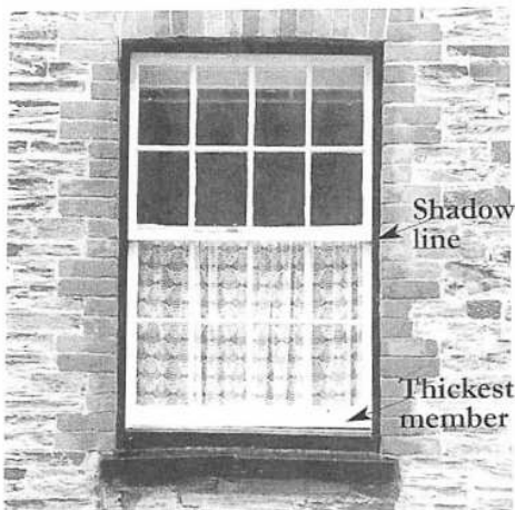
The real thing! A timber vertical sliding sash window. Note that the sides of the sash frames are wider than the central meeting rail and that the bottom row of the lower sash is the thickest of all. Note the shadow where the two sashes meet.
