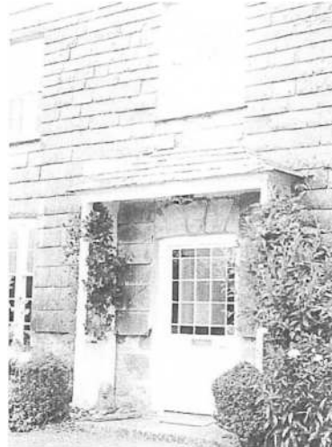
A Victorian door partly glazed with etched stained and cut glass panels. Retain these elements if at all possible.
