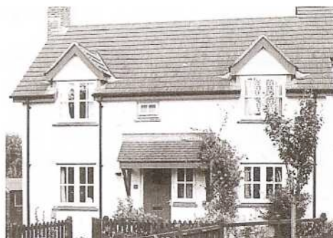
Modern cottage style house. The barge boards are rather too deep, but the overall effect successful.
