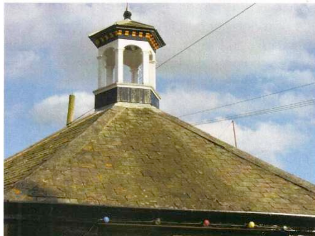
Fig 2: The Butter Market roof in West Looe
