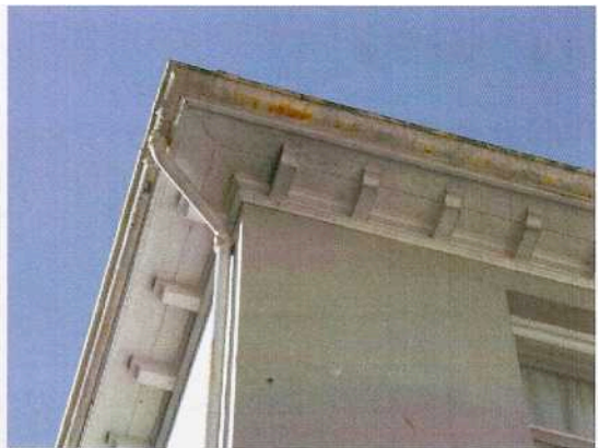
Fig 11: An overhanging bracketed eaves with boarded soffit
