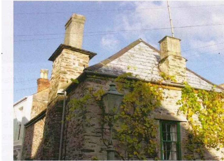
Fig 7: Tiled hips have a 'heavy' appearance compared with mitred hips
