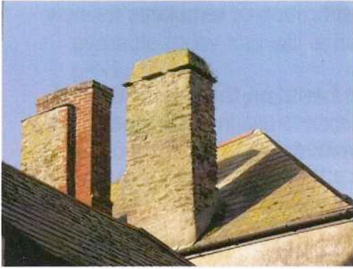
Fig 17: Chimneys add interest to roofscape and suggest phases of historical development
