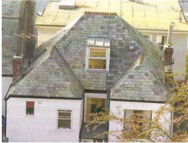
Fig 1: A U-plan roof in sized Delabole slate with mitred hips
