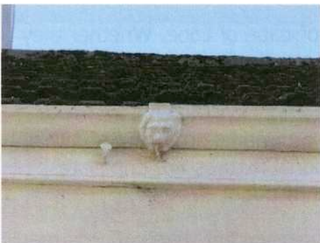
Fig 14: Lions heads on ogee gutters are relatively common in Looe
