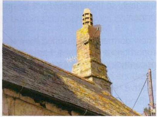
Fig 18: A traditional tapered stone stack with slate drips, later raised in brick with a functional pot
